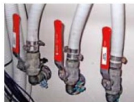
1998 boat built to RCD with non-marine brass valves
